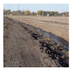
Silt fence, as shown in the detail drawings, must be installed properly to be effective. That means the bottom of the fence must be installed in a 6 inch deep trench and anchored with soil.
